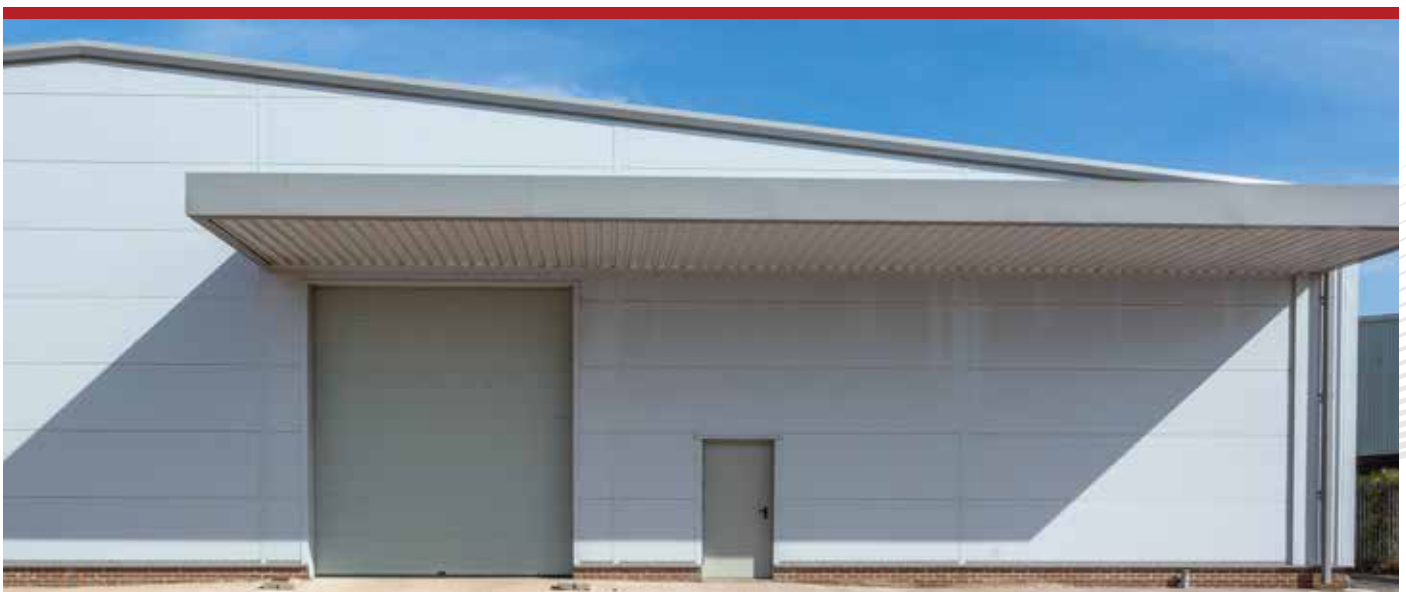
Canopy with soffit panels
